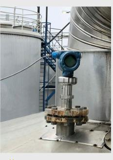
The Rosemount 5408 was able to handle turbulence. foam, and agitators and provide a reliable, stable level measurement. Perstorp Manager
